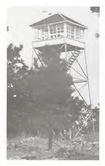
Figure 181. El Caso lookout, an Aermotor MC-24 on Quemado Ranger District.
